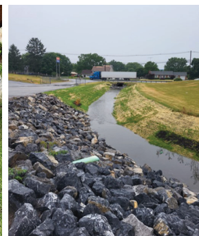
South Main Street Storm Water Best Management Practices Implementation
