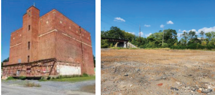
Site of Chambersburg Cold Storage Building before and after demolition.
