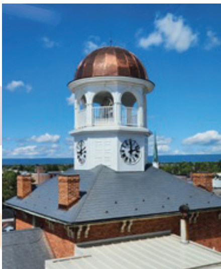
Fully Restored City Hall Cupola
