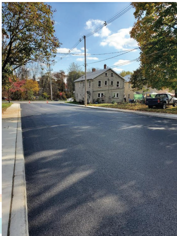
In 2023, Chambersburg finished the reconstruction of Center Street after three years of work.
